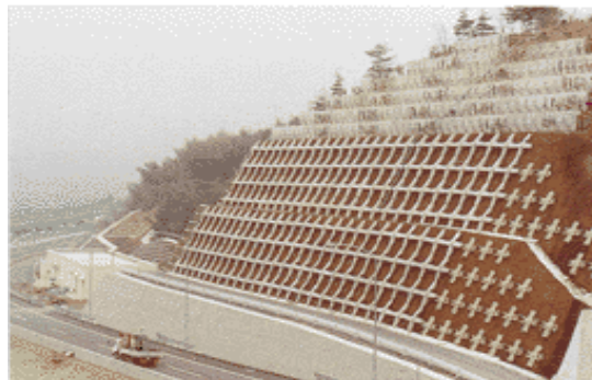
FIGURE 2.11 Use of Technora elements as ground anchors along the Meishin expressway, Japan [66]
