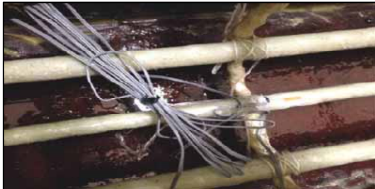
FIGURE 3.16 BFLA-5-5-3L applied on composite reinforcement
