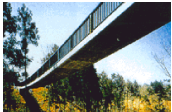
FIGURE 2.10 Use of CFRP bars in a stress ribbon bridge at the southern yard country club, Japan [66]
