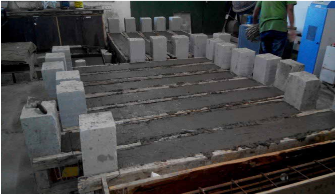
FIGURE 3.25 Beams after completion of concreting
