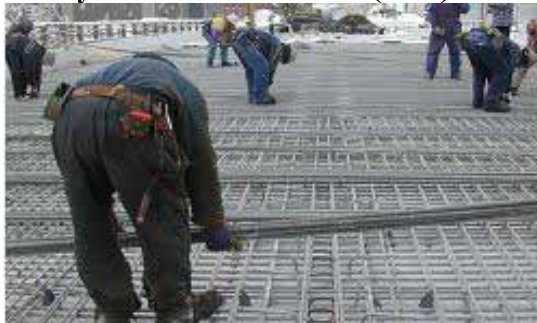
FIGURE 2.15 GFRP bridge deck, Cookshire-Eaton – Quebec [66]
