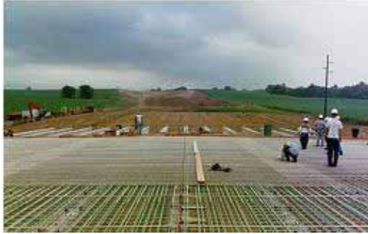
FIGURE 2.13 53 rd Ave bridge, city of Bettendorf – Iowa (USA) [66]
