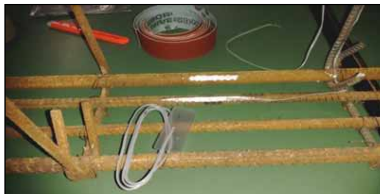
FIGURE 3.18 FLA-3-11-1L applied on concrete surface
