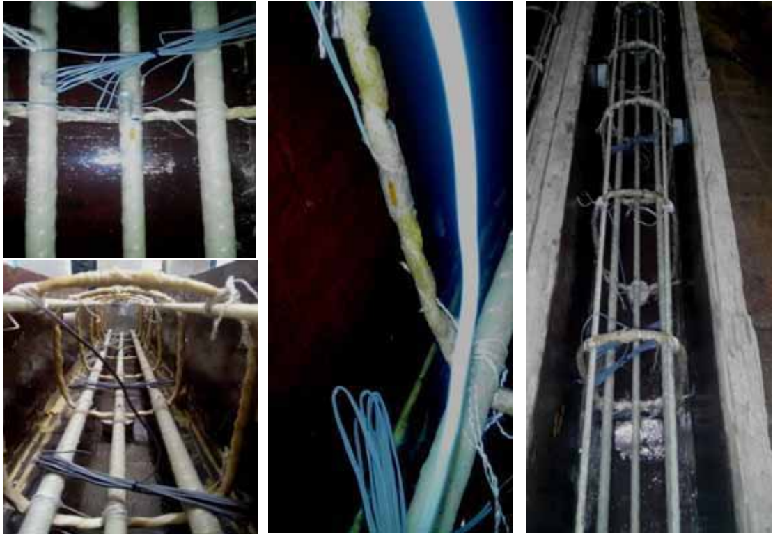
FIGURE 3.23 Application of strain gauge on longitudinal and shear reinforcement
