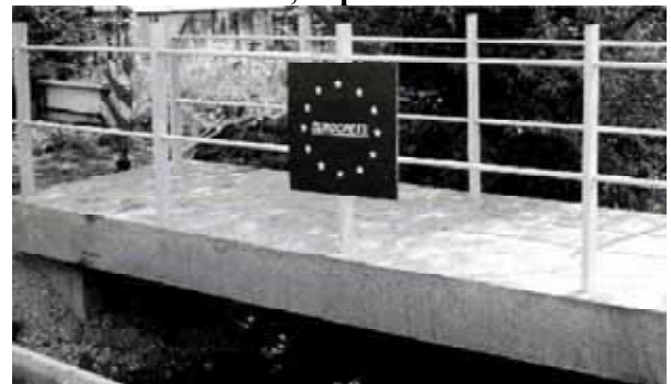
FIGURE 2.12 The first concrete footbridge in Europe with only FRP reinforcement (EUROCRETE Project) [66]
