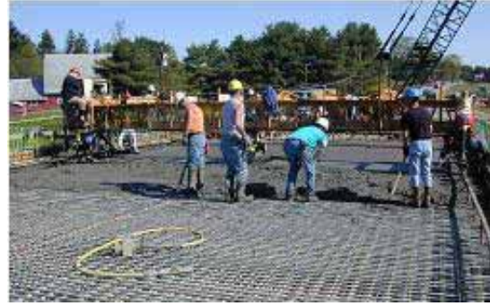
FIGURE 2.14 GFRP bridge deck, Morrystown – Vermont (USA) [66]
